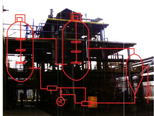
The selectivity for cyclohexene and the cyclohexene yield were stabilized at around 73% and 30%, respectively, in 419 h over a Ru-Co-B/ZrO<sub>2</sub> catalyst in a continuous device with two reactors in series.
