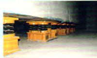
带基础块的弹性隔振系统 Spring vibration isolation system with foundation block
