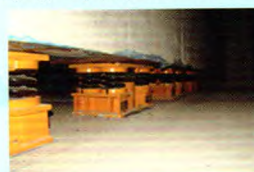
带基础块的弹性隔振系统 Spring vibration isolation system with foundation block
