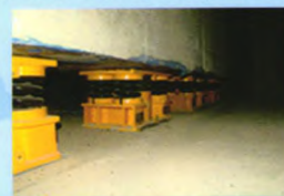
带基础块的弹性隔振系统 Spring vibration isolation system with foundation block
