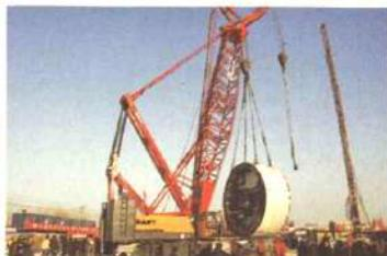
On Dec.28th, 2010, Sany SCC2500C crawler crane completed the suspension setting very well for 90t tunnel boring machine in Nanganqu item of South-to-North Water Transfer Project. SCC2500C adopted the special structure for the suspension setting of tunnel boring machine, namely, 19.5m boom and 7m fixed auxiliary boom. Sany specialized crawler crane brings about a turn for the suspension setting of tunnel boring machine from two cranes to only one.
