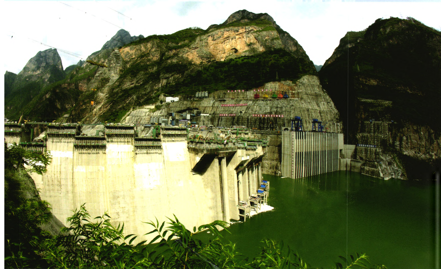
锦屏一级水电站大坝
