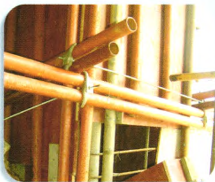
茂名石化钢柱加固
