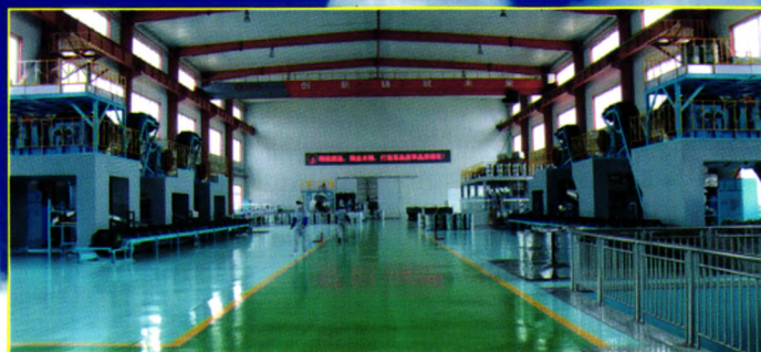
金达钛业精整车间 Finishing workshop
